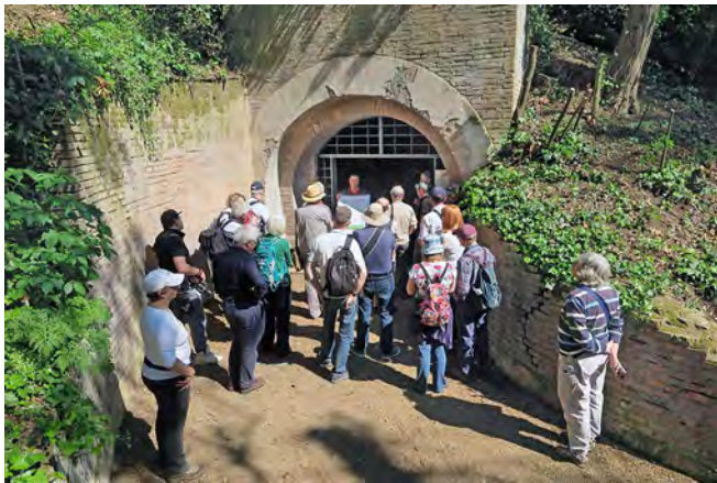
Surface briefing outside the Villa Ada shelter. The site was chosen for the small wooded hill above which gave both mechanical and visual protection
